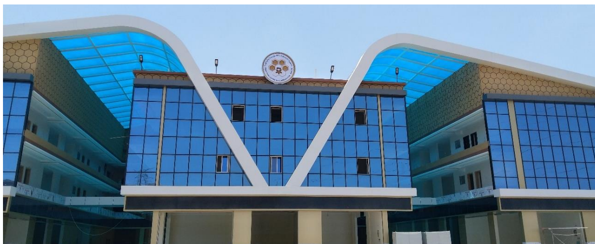
Figure 10: The new building under construction for the Beekeepers' Cooperative Association, Al Baha
