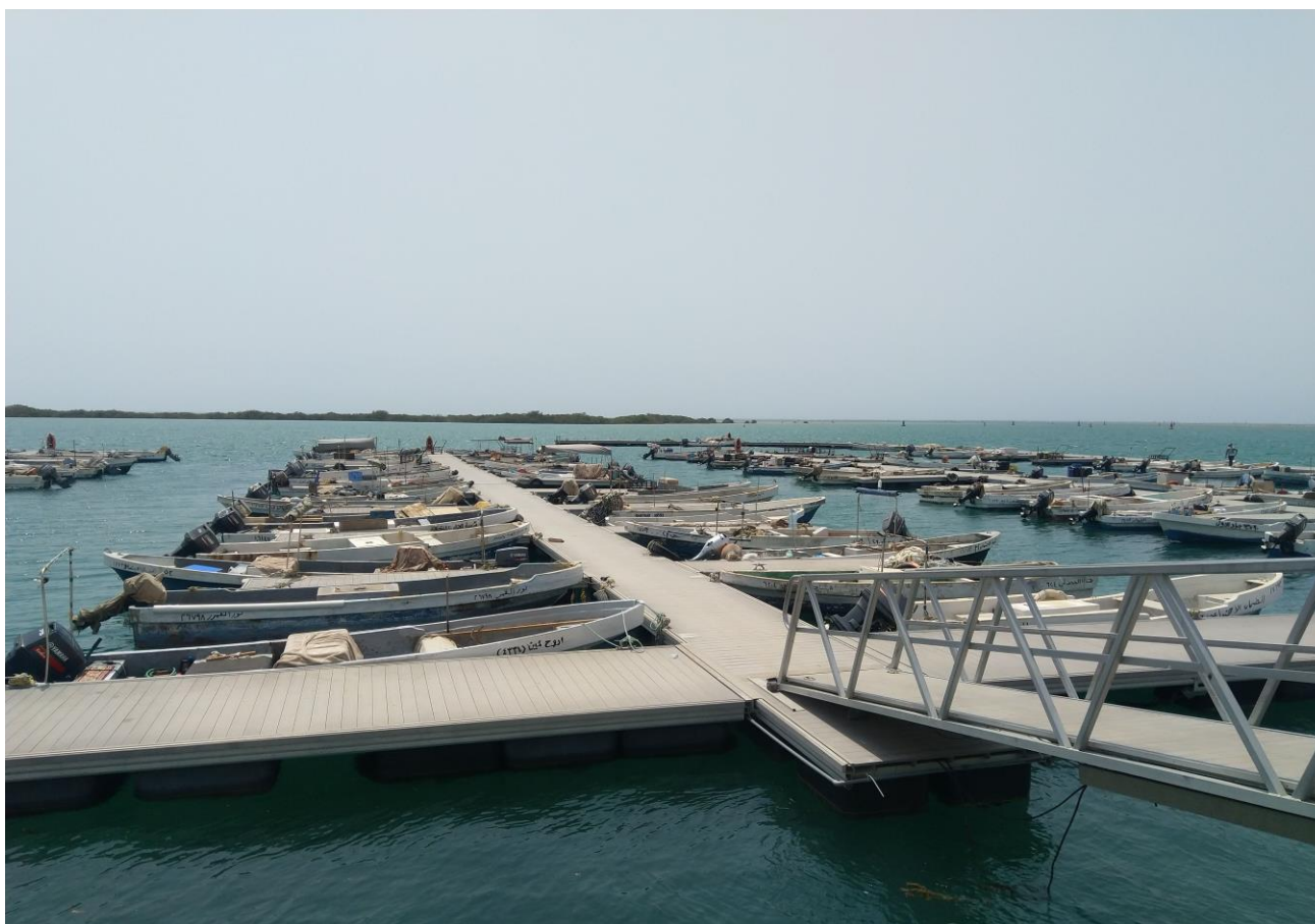
Figure 18: A Section of Thuwal Seaport
